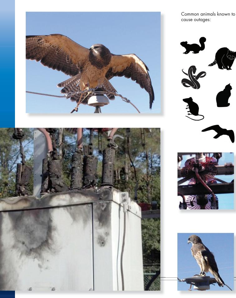
Damaged substation equipment caused by wildlife contact.
