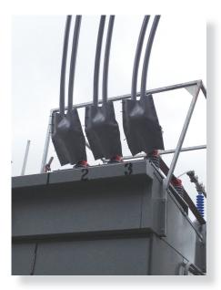
The E/Silicone Sheet is a high temperature vulcanized custom compound silicone sheet with a polyester fabric reinforcement. Made from 65 durometer silicone, almost 1/8" thick, it is a roll that allows you to custom cut covers for unique phase-to-phase and phase-to-ground areas of substation and distribution equipment.
